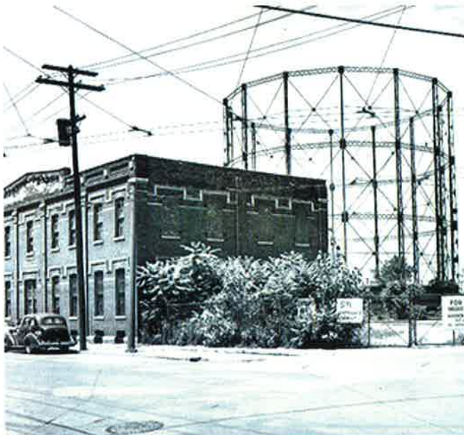
Example of Gas Holder at an MGP Facility
