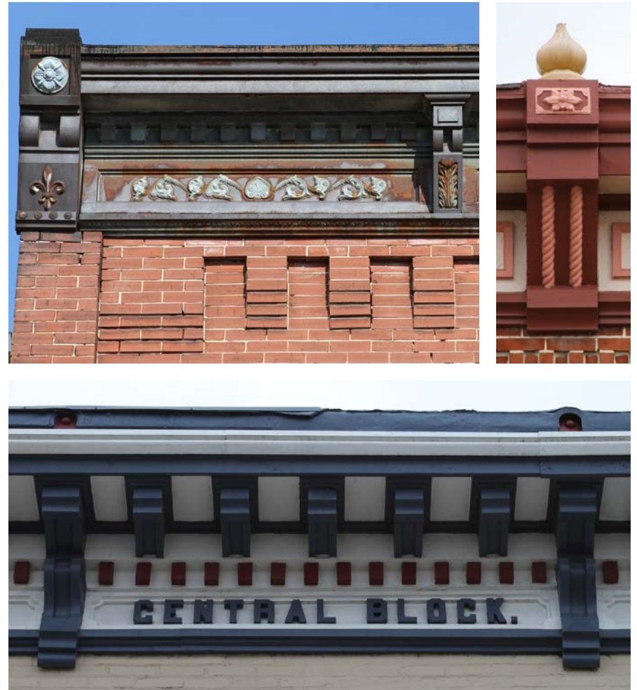
Cornice details giving character to Rochester downtown buildings include the decorative masonry craftsmanship and the pressed metal cornice at the wood panel and bracketed cornice at 530 Main (upper left), 727 Main (upper right) and 724-726 Main (lower).
