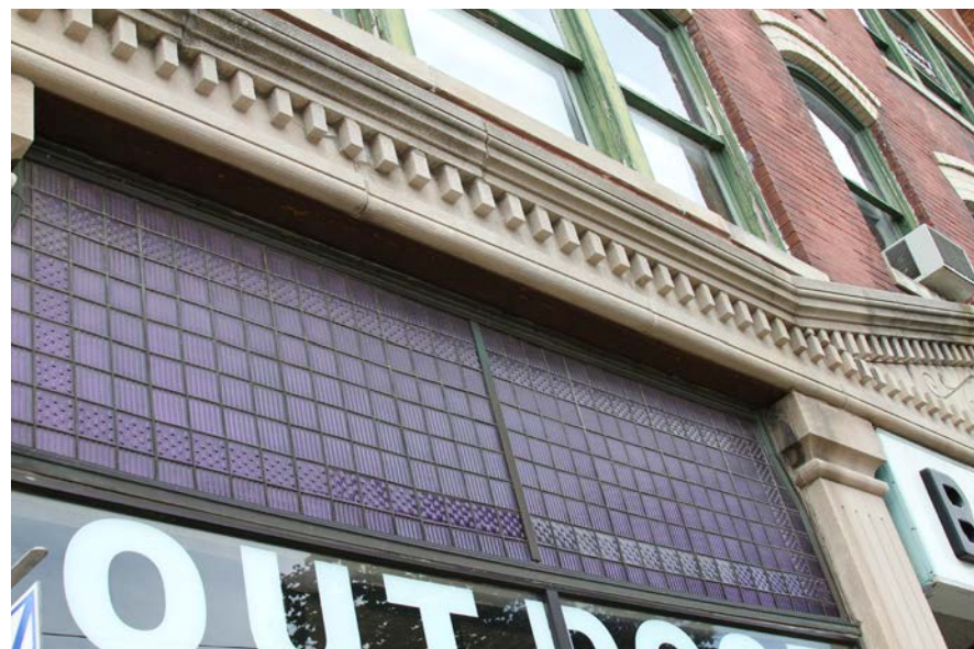
Dentil cornice on the Dillon Building.
