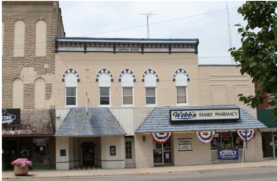
The Italianate style expressed in the Central Block includes the bracketed cornice and decorative window hoods.
