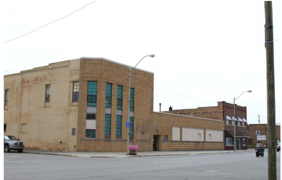
The angled corner and ribbon windows on the Brackett Building illustrate the Art Moderne style.
