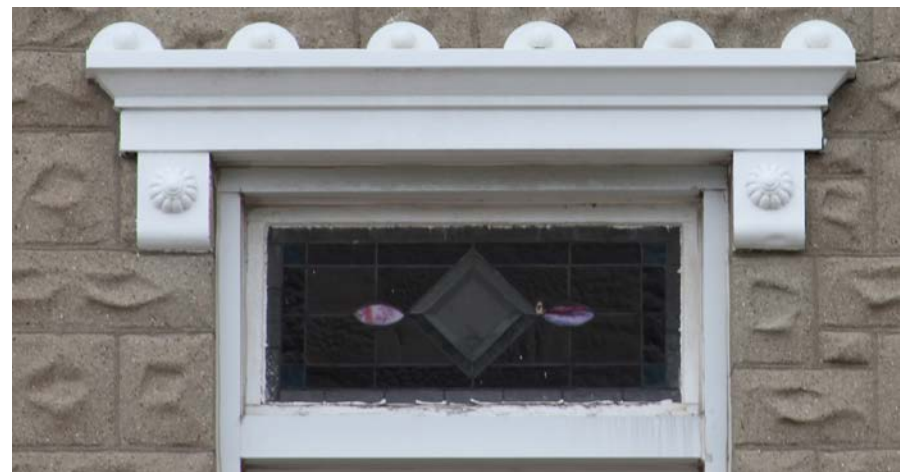
Masonry pediment with limestone medallion with symbol of Caduceus, above and metal window hood topping a leaded-glass transom window below.
