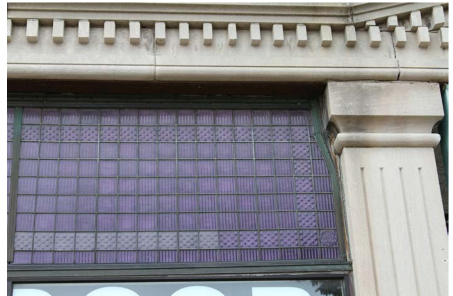
The prism glass transom at 712 Main allowed light to filter deep into the store.
