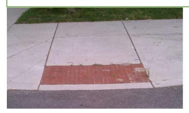
Grade B – Minor Deficiency: The ramp shown has no detectable warning.
