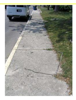
Grade D – Multiple Major Deficiencies: For instance, the sidewalks shown here are too narrow, they have joint displacements, rough/cracked surfaces, and gaps making it likely impassable by wheelchair, though a fit walker could still navigate the sidewalk.
