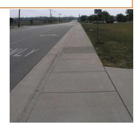
Grade C – Major Deficiency: For instance, the sidewalk shown here is too narrow and has joint displacements making it complicated to navigate by wheelchair, though still passable for someone walking.
