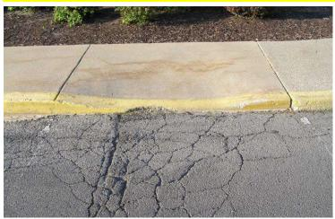
Grade D – Multiple Major Deficiencies: The ramp shown here is too narrow, is too steep, has a bad cross slope, and no detectable warning.
