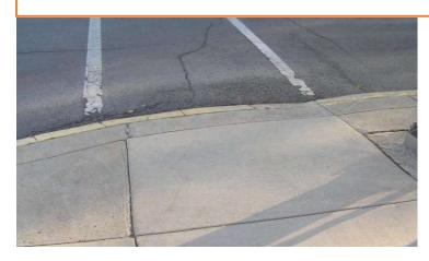
Grade C – Major Deficiency: The ramp shown here is too narrow, doesn't have a detectable warning, and has a joint displacement.
